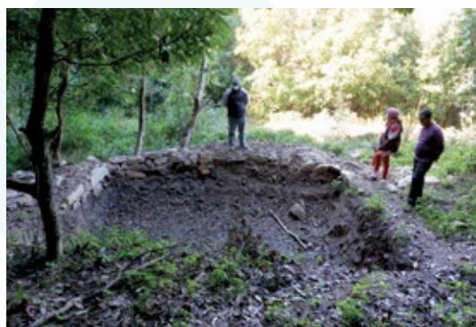
Recharge pits and ponds for natural groundwater percolation to overcome water scarcity.
