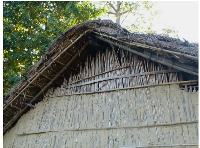
Fig. 7. Gable opening for air circulation in Tharu House, Chitwan.
