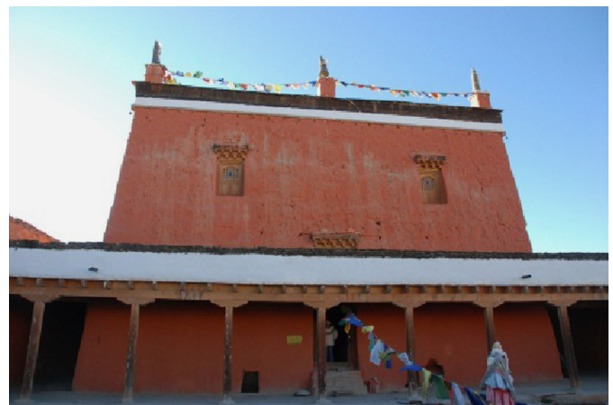
Fig. 16. Typical small windows in building façade in Upper Mustang.
