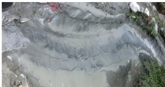
Fig. 6 Highly silted irrigation infrastructure in the Trans-Himalaya, Nepal
